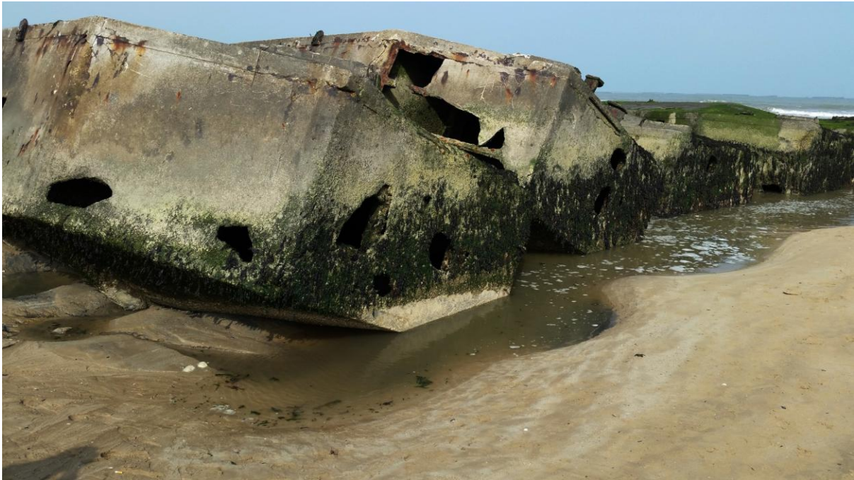
Figure 59 More Mulberry remains, this time concrete 'Beetles' - floats used in the construction of a roadway to the pier heads (Whale). Again we came across a number of these in our Mulberry 70 project. (Martin Davies)
