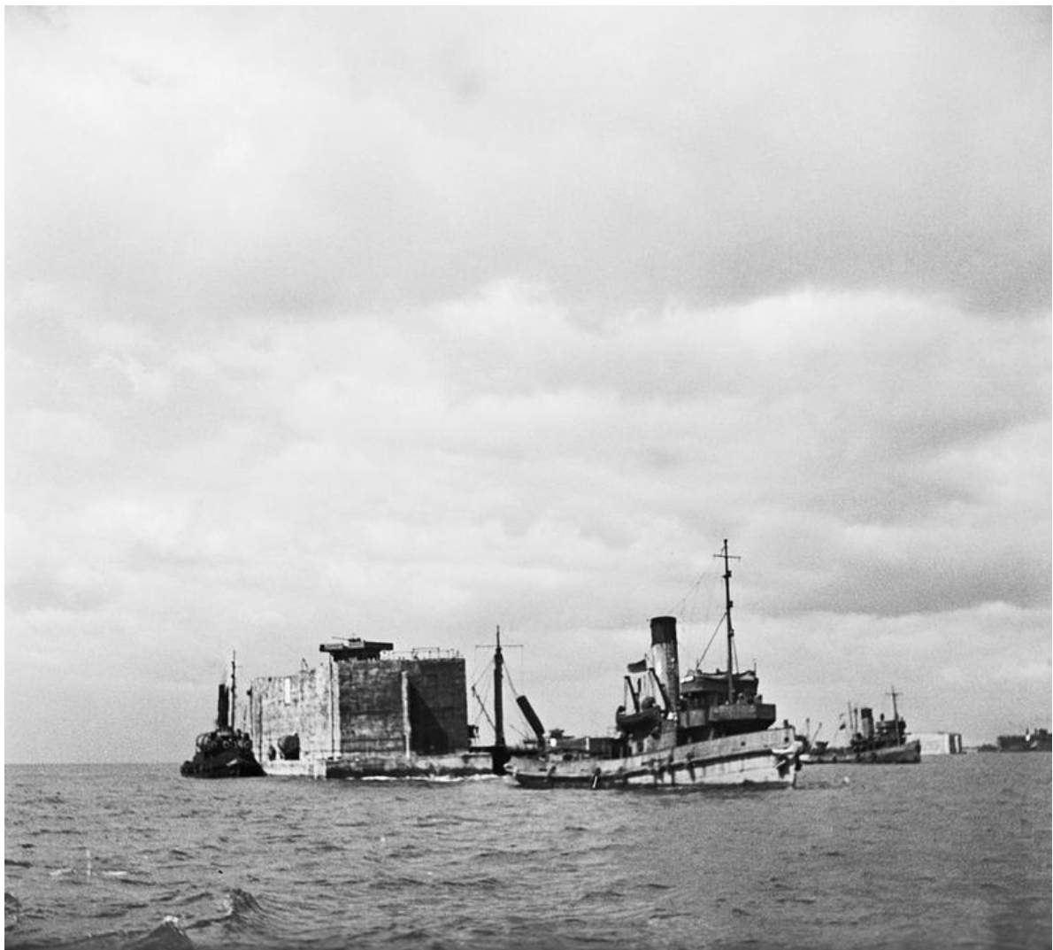
Figure 16 A Mulberry Harbour Phoenix A unit under tow across the English Channel. Note the Bofors gun on the top. © IWM (H 39300)
