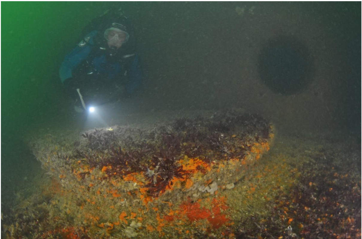
Figure 24 One of the towing point for the Phoenix Unit. (Martin Davies)
