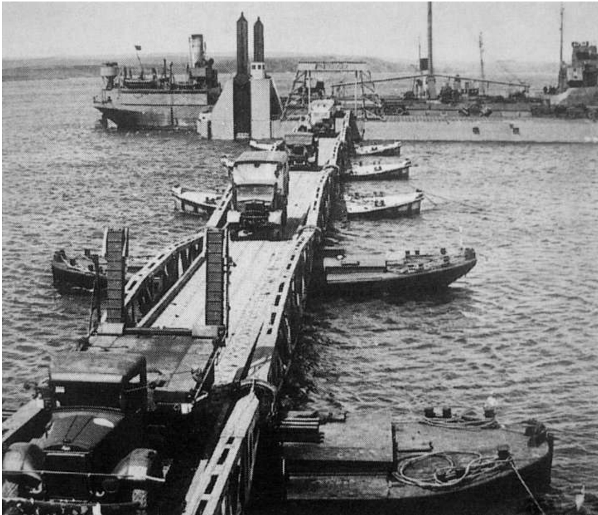
Figure 73 - Whale Bridge and supporting 'Beetles'.
