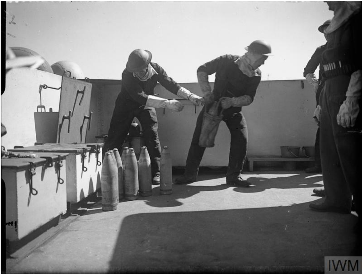
Figure 20. Passing 4.7 inch projectiles through the hatch of a Landing Craft Gun (Large) (LCG (L)) during an invasion rehearsal off the Isle of Wight. Note the crew wearing anti-flash clothing. (© IWM A 23771)
