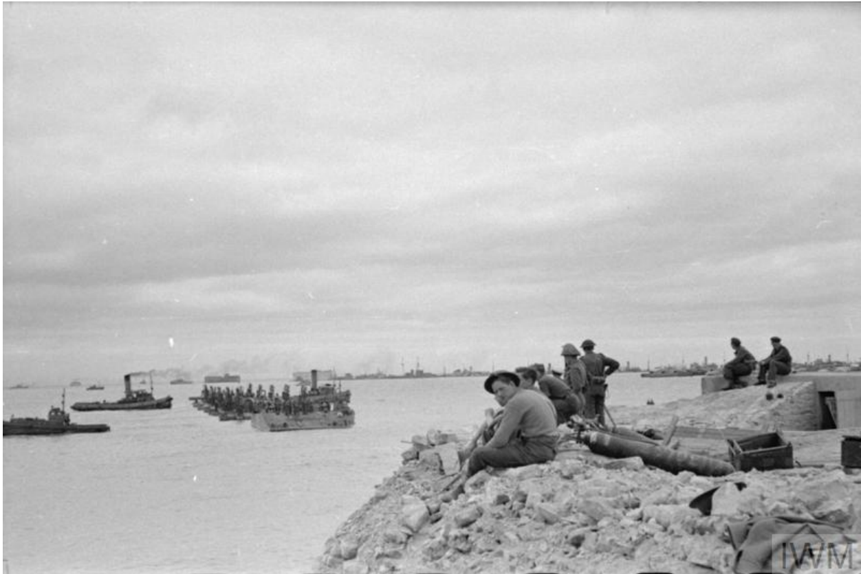
Figure 87 Mulberry Harbour, Arromanches: A section of a "Whale" is being towed into position. In the foreground men are sat on the shore watching the construction of the harbour. (© IWM (A 24157))
