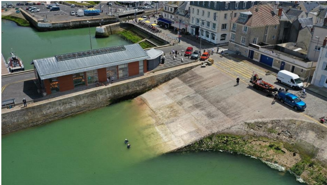
Figure 8 the launch site at Port-en-Bessin. (© Martin Davies)
